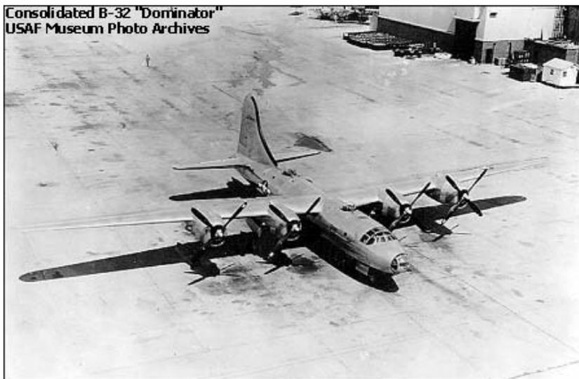
B-32 42-108471, the first production aircraft, seen fitted with a single B-29 fin. Note also the revised cockpit and nose layout. (USAF Museum)
